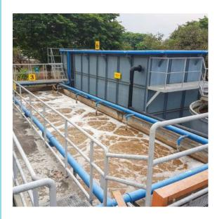
At MHRIL resorts, nearly 80% of wastewater originates from showers and washbasins. When treated separately from black water, this greywater achieves up to 90% recovery, translating into significant gains in water efficiency and cost savings.
